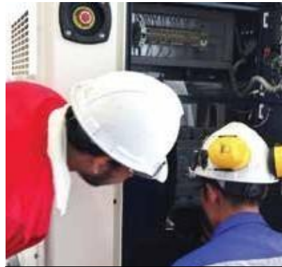
Support Genset Rumah Sakit
